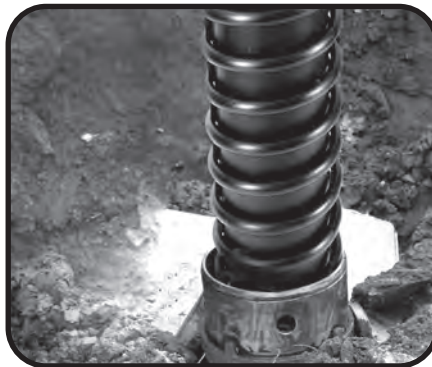
Inserting of VTP® in the borehole with hollow stem auger
