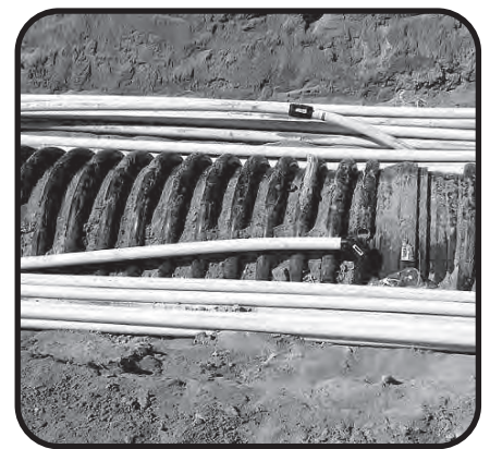
Easy connection of connection pipe via electro fusion coupler
